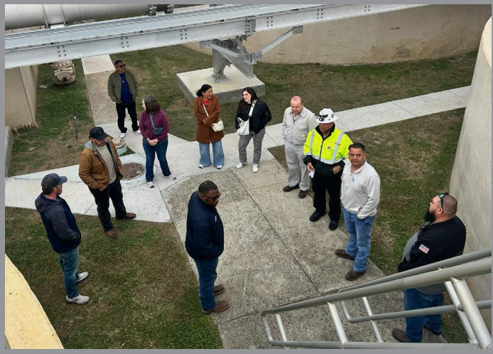
Gathering the group - how the processes work get a solid understanding of the treatment processes.
