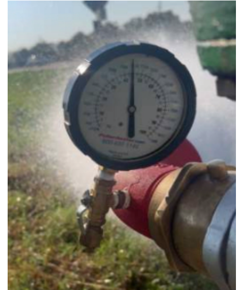
Fire flow testing Images
